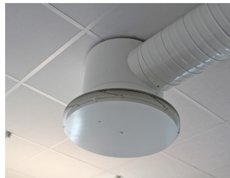
Visible mounting of the active supply air diffuser TTC with plenum box HTR.
