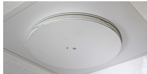
An active supply air diffuser mounted with cover plate UTD in place.
